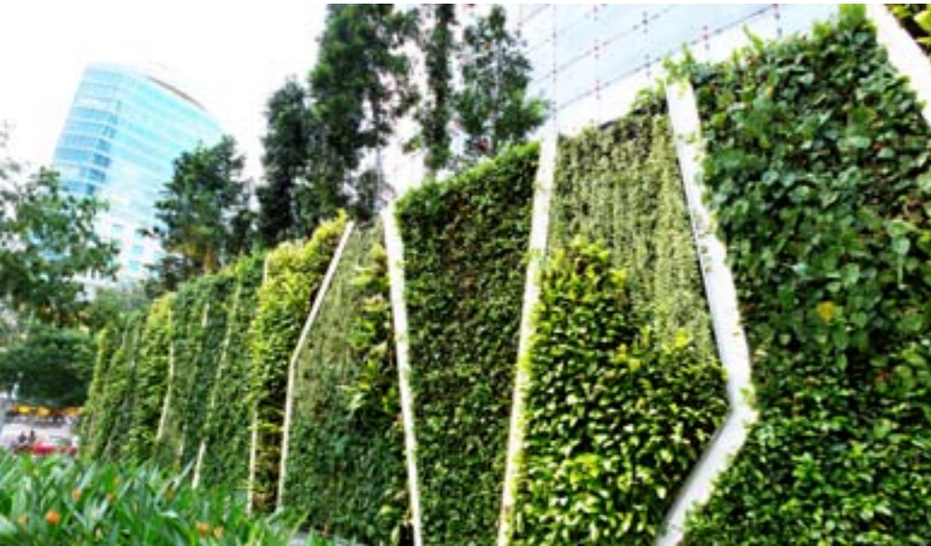
Lush greenery punctuates the walkways along Paterson Road and Orchard Boulevard. A verdant vertical wall, spanning 60m in length and 3m in height, lines the building along Orchard Road. To enhance this vertical garden, shards of stainless steel troughs are used, adding a touch of randomness, and punctuate the evening with a symphony of lights.
